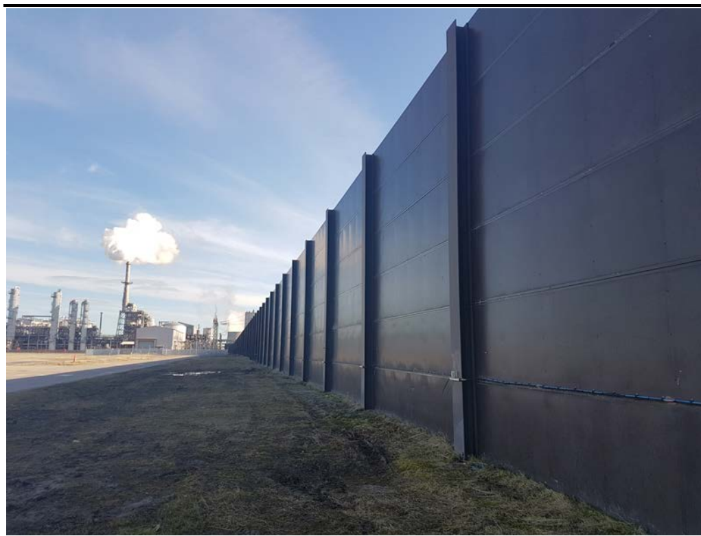
Figure 5.2 Existing Southern Noise Control Wall
